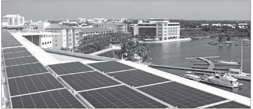
Dart Realty and Cayman Solar installed 302 photovoltaic panels that produce 76 kilowatts of renewable energy at 89 Nexus Way in Camana Bay.
